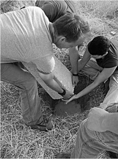
The Zincirli Expedition team placing a concrete survey marker on the site during the 2006 season. Seventeen survey markers were placed on and around the site and their precise locations — accurate to one centimeter horizontally or vertically — were determined using GPS satellite readings
