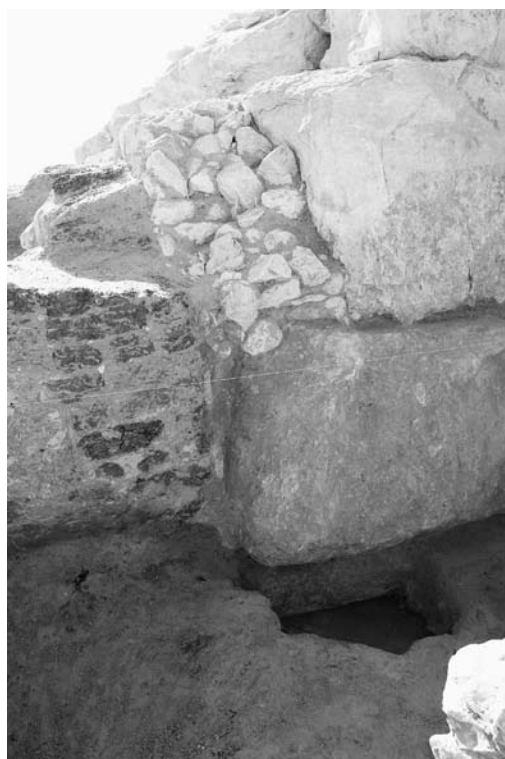
Figure 11. WCNE juncture at the foundation of the Wall of the Crow. Note foundation slab beneath the corner stone of the Wall of the Crow. View to the southwest
