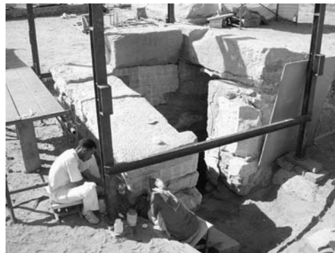
Figure 7. The southern well being consolidated by conservators Mohamed and Nehal. Photo by Ray Johnson
