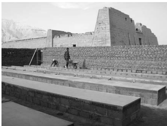
Figure 8. New Medinet Habu blockyard under construction. Photo by Ray Johnson
