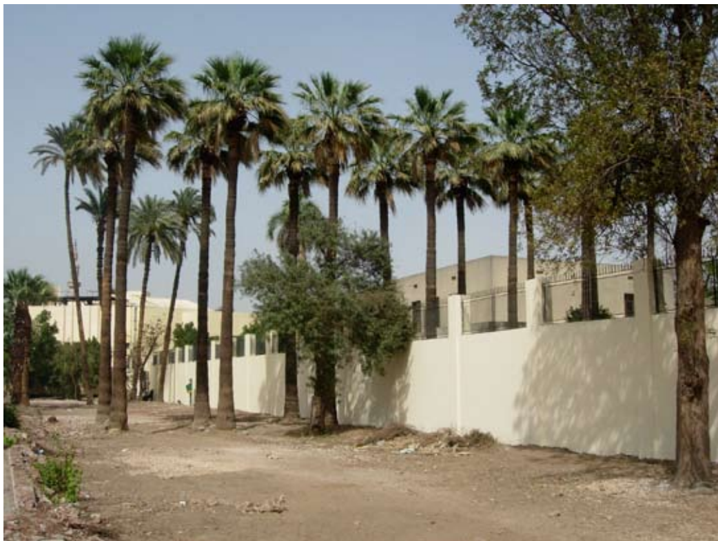
Figure 16. Chicago House, new front wall, April 2009. Photo by Ray Johnson
