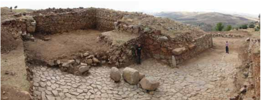
Figure 8. Photograph of the inside of the gate passage and chamber showing the extent of this year's excavation. Excavation will continue next year with the removal of the remaining portion of collapse in the gate chamber
