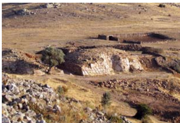
Figure 6. A view of the outside of the Cappadocia Gate showing the preserved sloping stone glacis that once stood at the base of the external walls and towers. The new walkway created to the east of the gate to divert animal traffic around the gate passage can be seen on the right of the photograph
