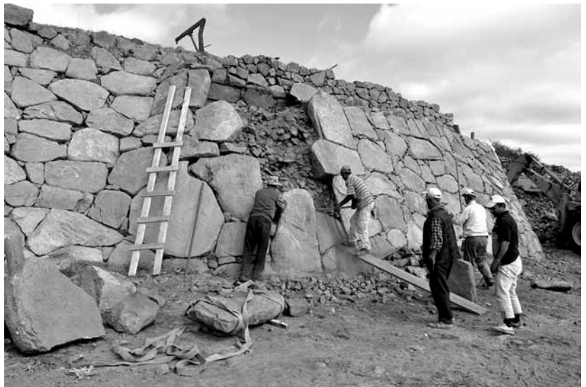
Figure 17. Reconstruction of the Cappadocia Gate glacis in progress
