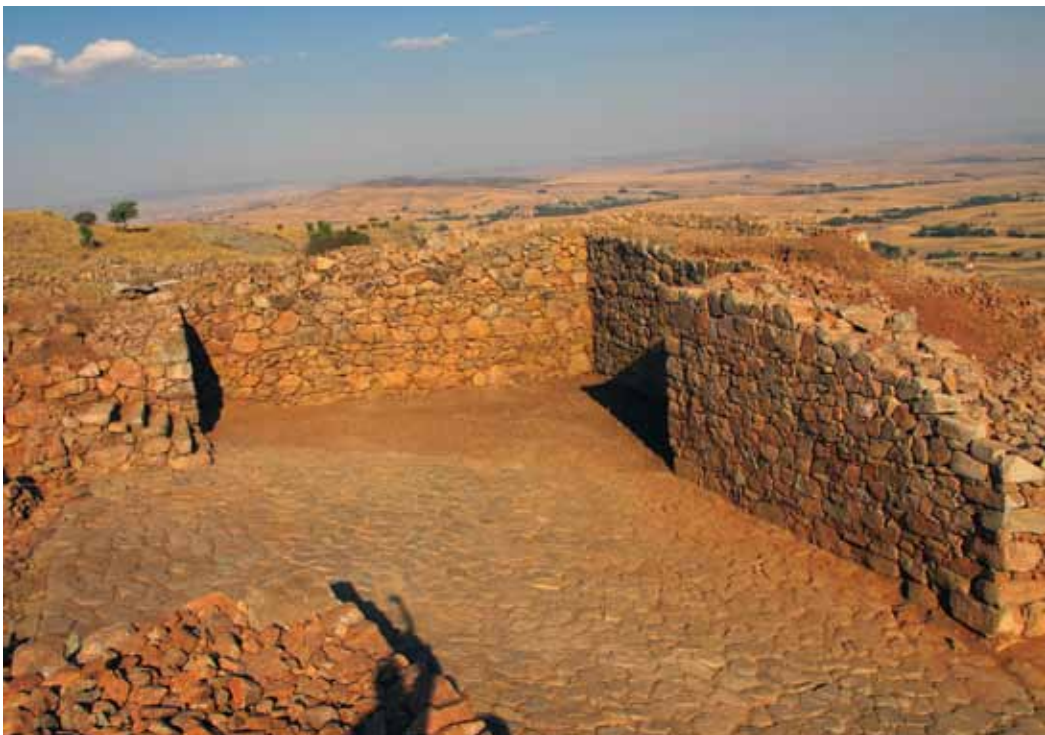
Figure 16. The central court of the Cappadocia Gate following restoration efforts on the three towers
