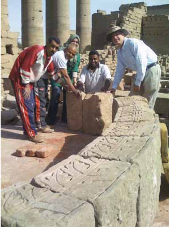
Figure 9. Sayid, Mohamed, MSA Inspector Marwa Abdel-Naby, Saoud, and Jay joining Thecla Church arch blocks. March 14
