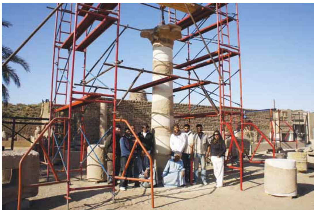
Figure 3. Re-erected column and Medinet Habu conservation team. January 27
