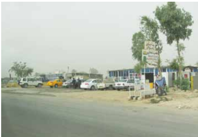
Restaurant encroaching on super highway south of Baghdad
