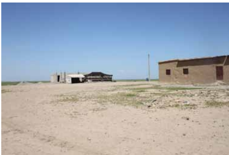
Figure 3. Hamoukar, April 2012: illegal building next to dig house
