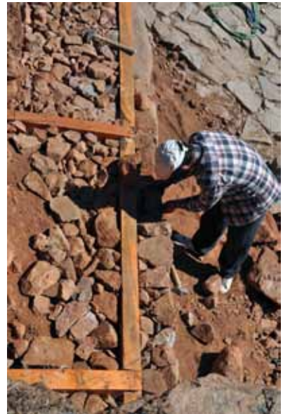
Figure 15. Restoration efforts of the North and West Towers involved incorporation of new wooden beams behind the facing stones in order to replace the beams that burned out in the final destruction of the city
