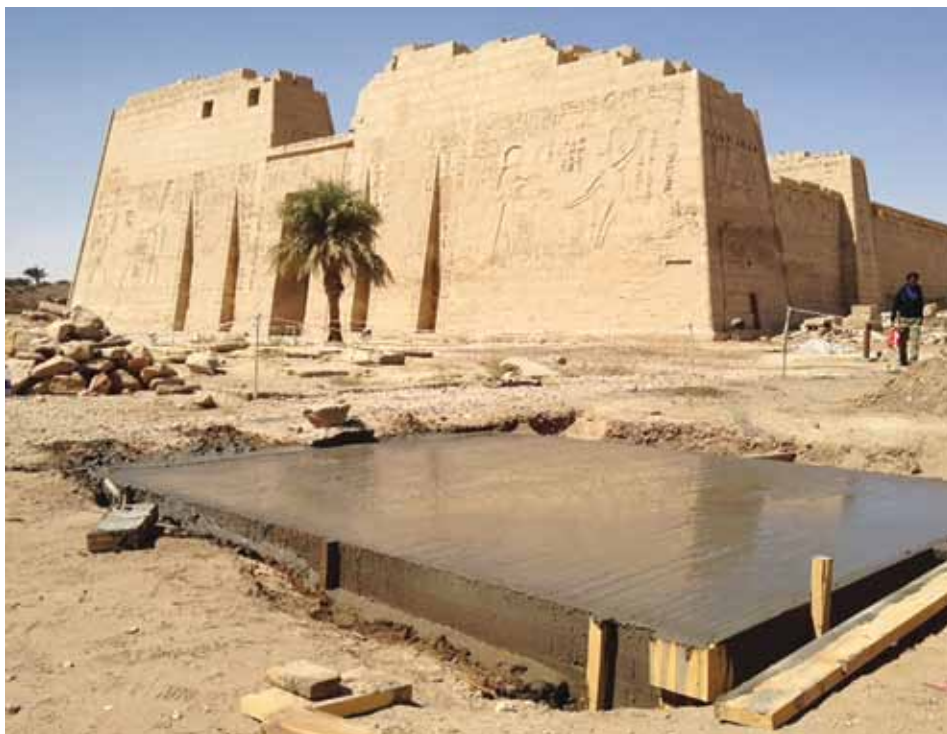
Figure 5. Poured, reinforced-concrete foundation for the Domitian gate. Medinet Habu. Photo by Frank Helmholz
