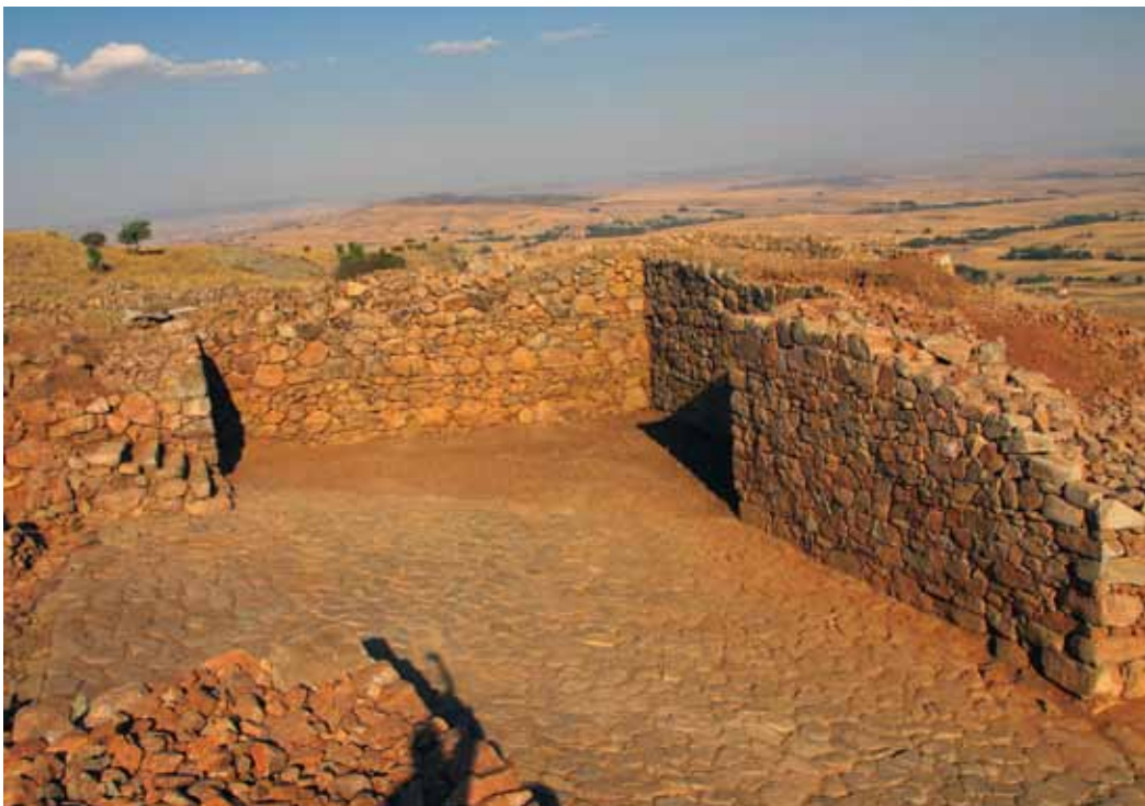
Figure 16. The central court of the Cappadocia Gate following restoration efforts on the three towers
