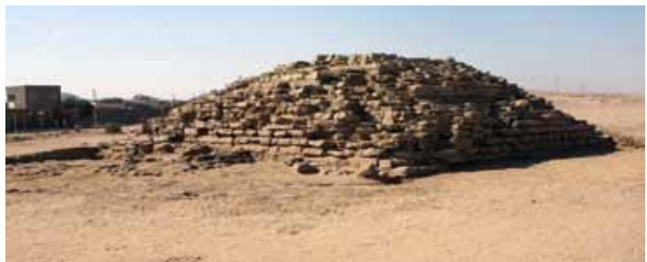
Figure 3. Eastern face after cleaning
