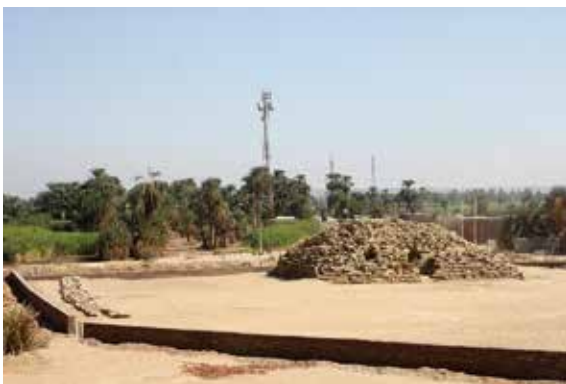
Figure 19. The new wall protecting the pyramid site, view to the southeast
