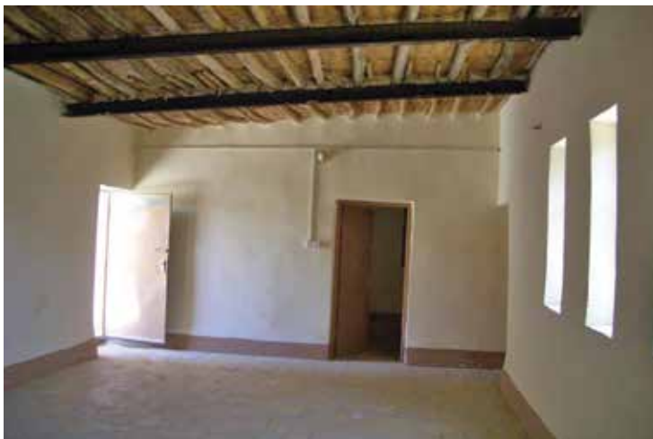
Workroom burned in 1996, new roof and electricity
