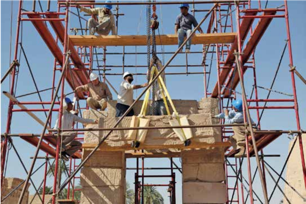
Figure 8. Medinet Habu Domitian Gate cornice raising, March 22, 2015 (photo: Yarko Kobylecky)
