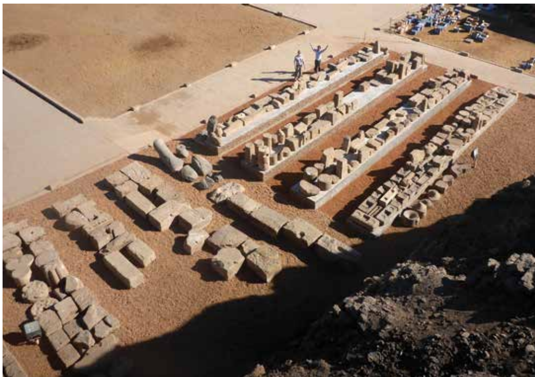
Figure 15. The Edfu blockyard area with the platforms at the end of the season
