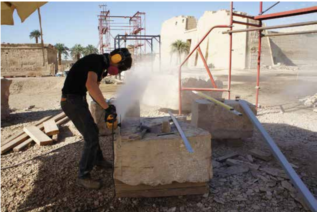
Figure 1. Johannes shaping stone for the Domitian Gate restoration, Medinet Habu (photo: Ray Johnson)
