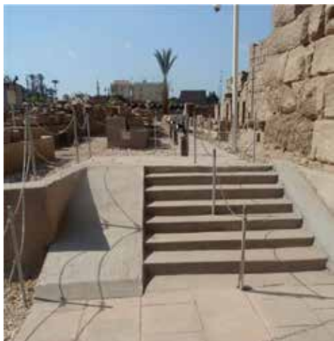
Figure 21. The new access ramp (photo: Ray Johnson)
