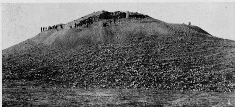
Excavating the Citadel Wall Encircling the Summit of the Alishar Mound
