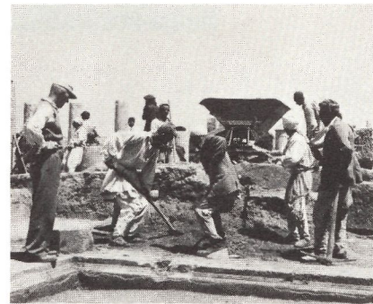
Excavations at Tolmeita, Libya
