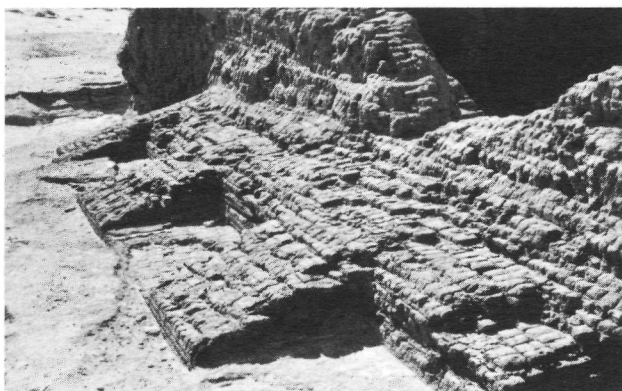
Bases of butresses of the east wall of the fortress at Serra East
