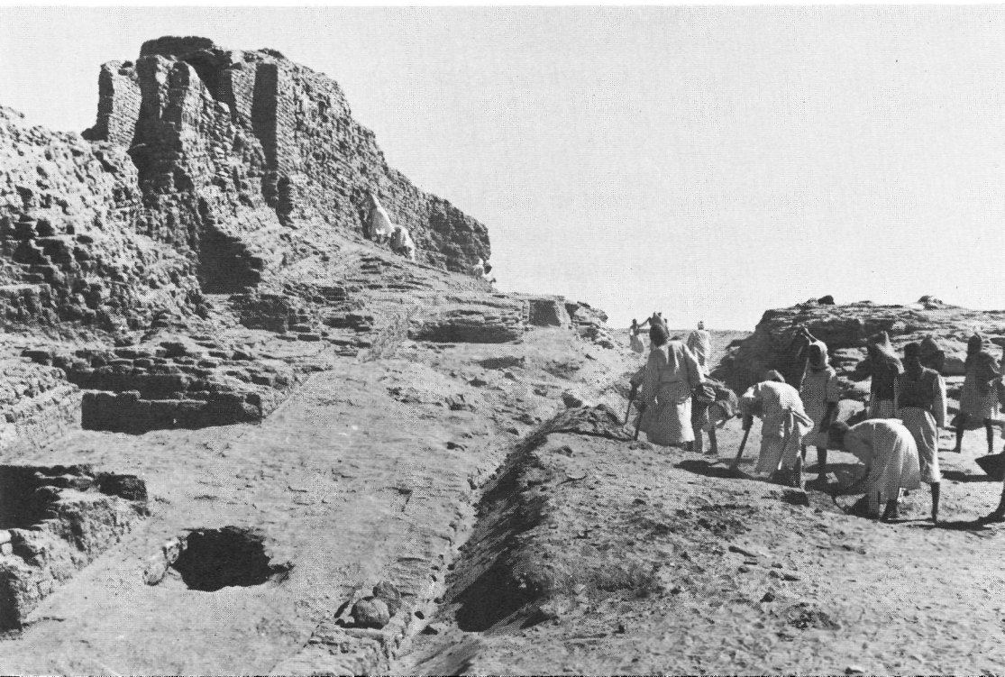
Clearing fosse on south side of fortress at Serra East in Nubia
