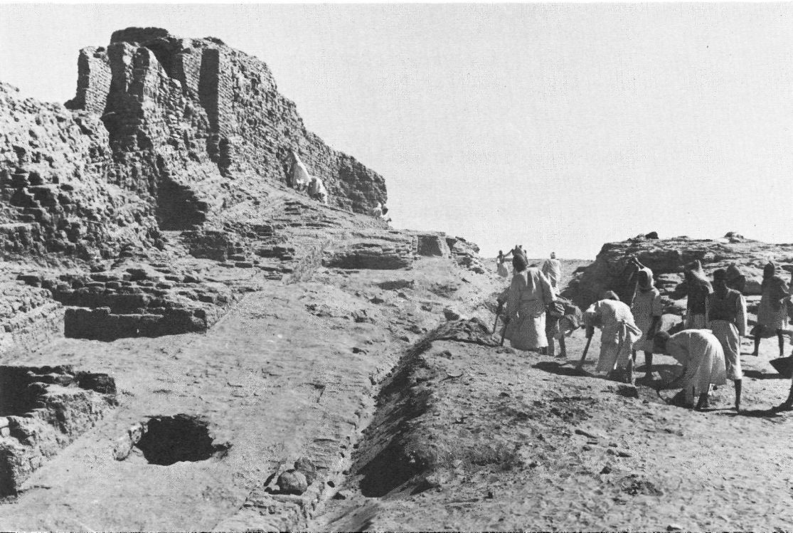
Clearing fosse on south side of fortress at Serra East in Nubia
