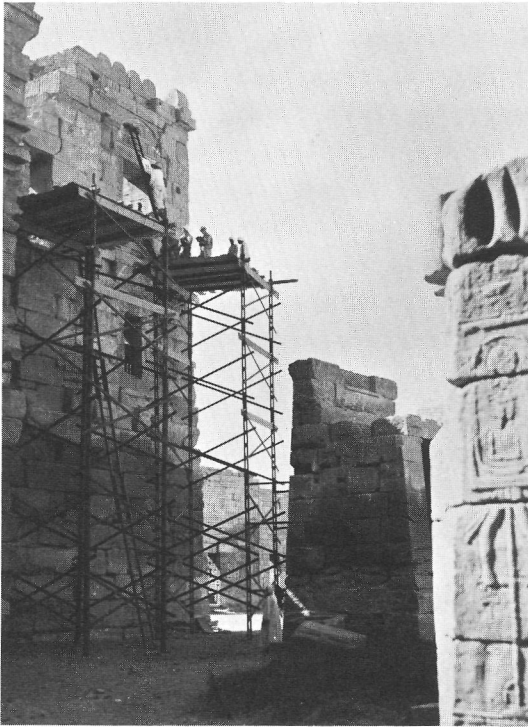
Work at the High Gate, Medinet Habu.
