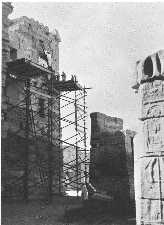
Work at the High Gate, Medinet Habu.
