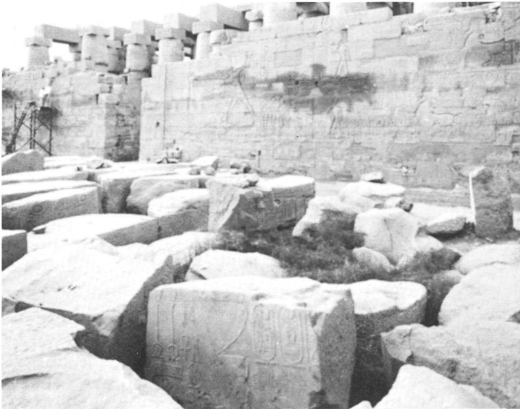
General view of the north wall of the Hypostyle Hall at Karnak, where Chicago House staff members are now recording the important historical reliefs of Seti I. Photo by John Ross
