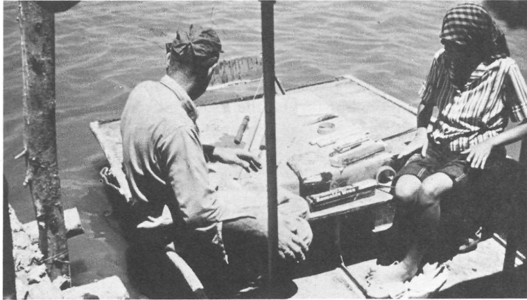
The tool used in coring, and some palynological samples wrapped in aluminum foil to preserve them. Photographs from another of H. E. Wright's expeditions, at Houleh, Israel.
