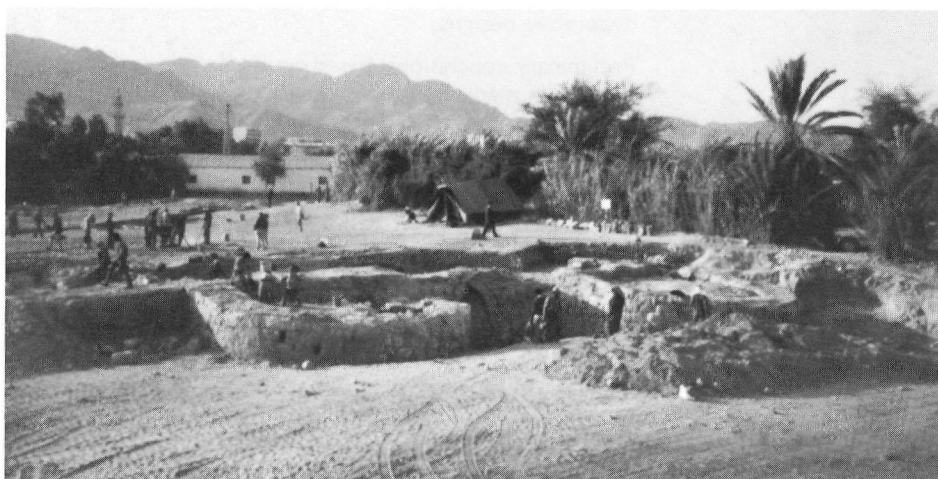
● Aqaba: City wall with towers and gateway.
