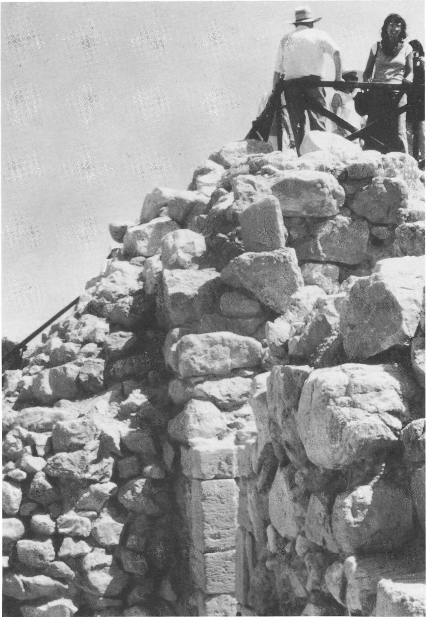
Detail of the Khirbet Qumran tower; note the buttressing ramp of boulders and the fine stonework of the original vertical structure
