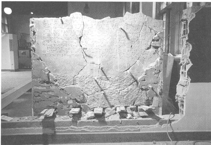
The first inscription discovered on the back of OIM A7365. The wall has been removed from the back of the relief, exposing the metal L-shaped ties that held the stone pieces to it. At periodic intervals, bricks of the plinth beneath the relief have been removed to allow the insertion of metal plates that will be used to lift the relief. Until the relief is lifted, wooden shingles inserted in the holes provide support for the stone above
