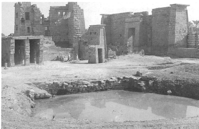
Figure 1. General view, from the northwest, of the small temple of Amun at Medinet Habu and its sacred lake; the eastern High Gate looms behind
