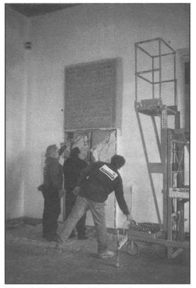
Figure 1. Doug Mertes, Milt Samuelson, and Bill Allison, Sr., from Belding/Walbridge preparing to remove an inscribed glazed brick panel from wall in order to relocate it as part of the Persian Gallery reinstallation. Photograph by Laura D'Alessandro
