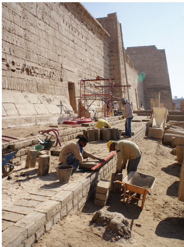
Brick laying in southern sector. Medinet Habu. December 16, 2016. Photo by Ray Johnson
