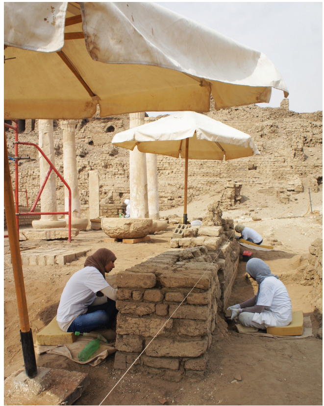
Butehamun House brick restoration. Medinet Habu. Photo by Ray Johnson
