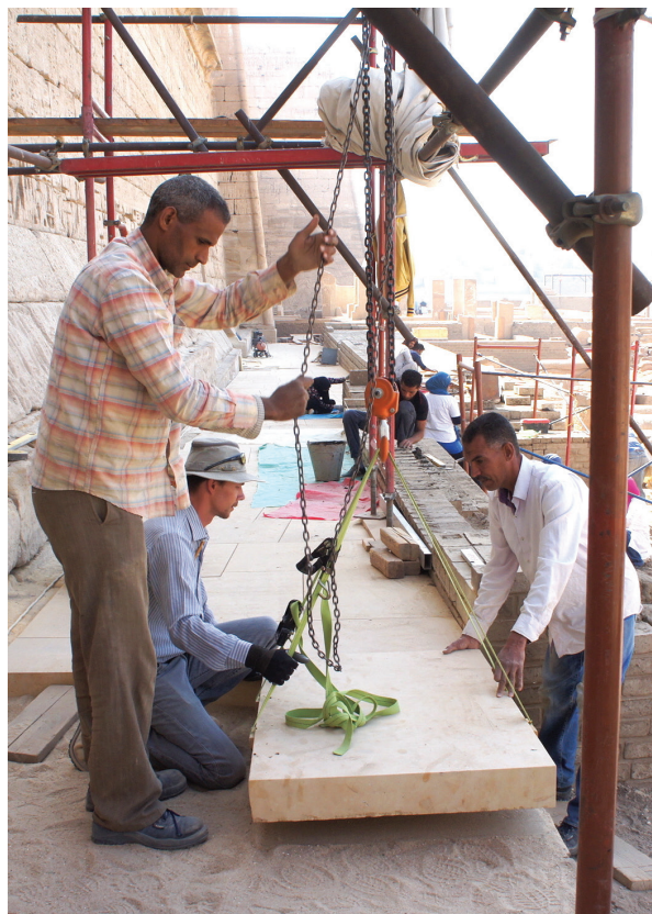
Laying new paving at Medinet Habu. March 29, 2017. Photo by Ray Johnson
