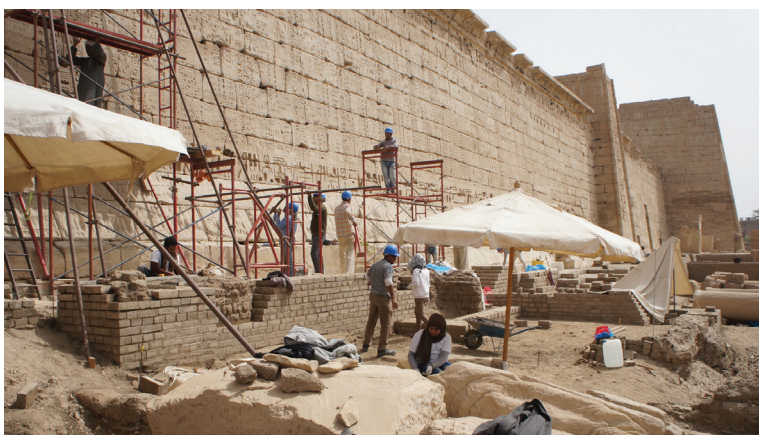
USAID-funded restoration work on southern area. Medinet Habu. February 22, 2017. Photo by Ray Johnson
