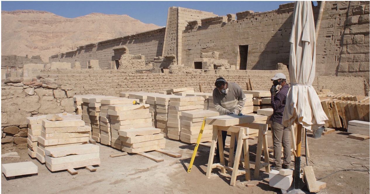
Mohamed and brother Mahmoud shaping sandstone slabs for the southern walkway. Medinet Habu. Photo by Ray Johnson
