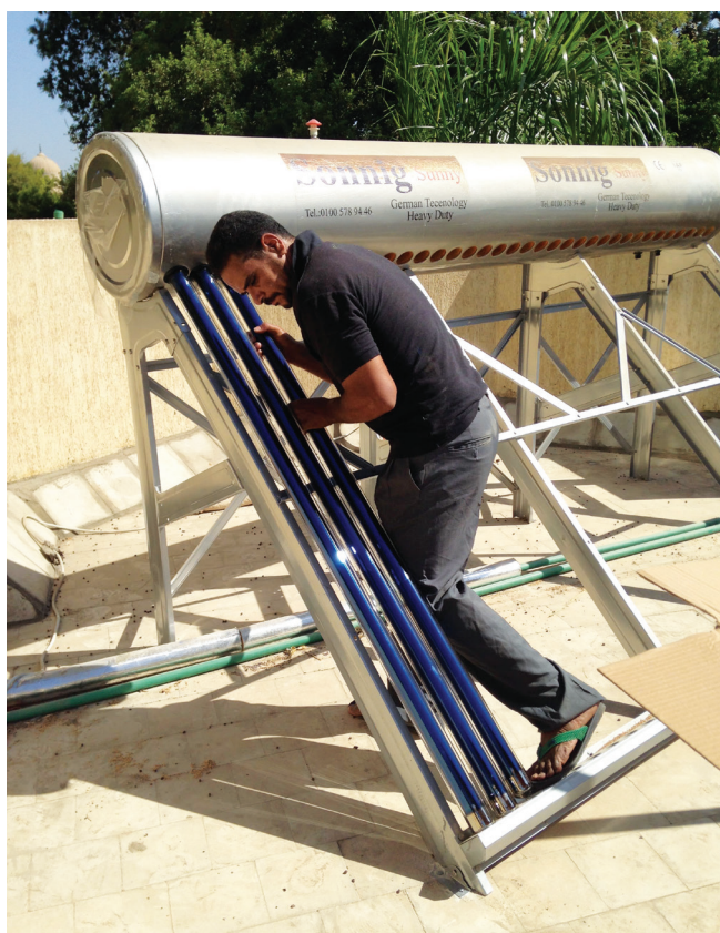
Installation of solar water heaters over Healey House. Chicago House. September 2016. Photo by Tina Di Cerbo
