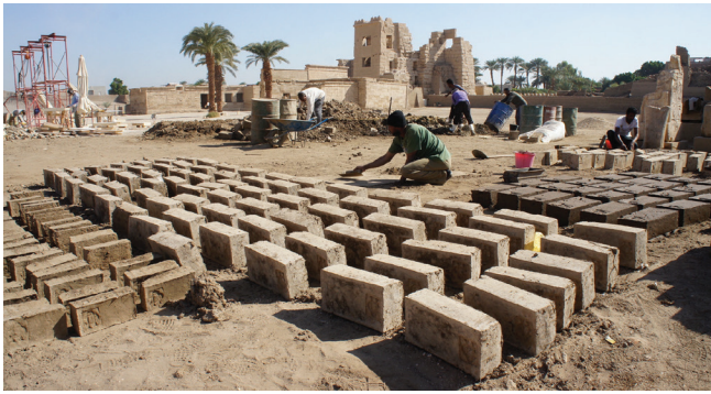
Brickmaking. Medinet Habu. December 16, 2016. Photo by Ray Johnson
