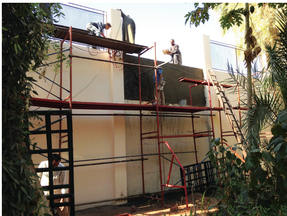
Southern wall raising. Chicago House. Photo by Tina Di Cerbo
