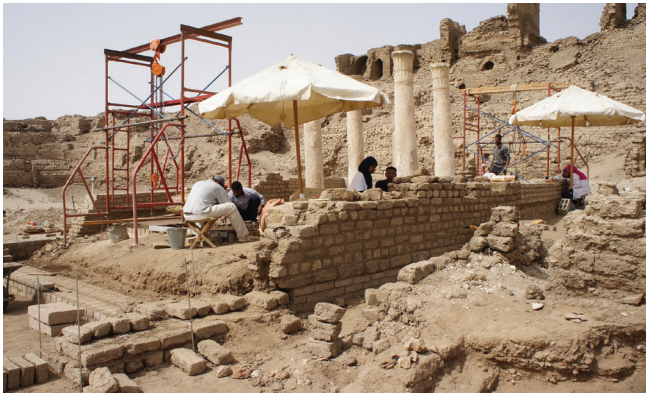
Butehamun House restoration work. Medinet Habu. Photo by Ray Johnson
