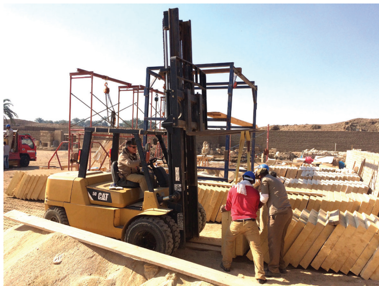
Frank using forklift to move stone slabs for restoration. Medinet Habu. February 7, 2017. Photo by Johannes Weninger
