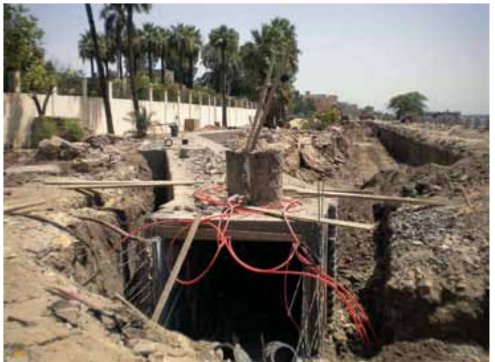
Corniche service tunnel and riverbank construction, June 2010
