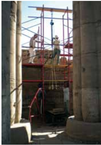
Amenhotep III wall construction
