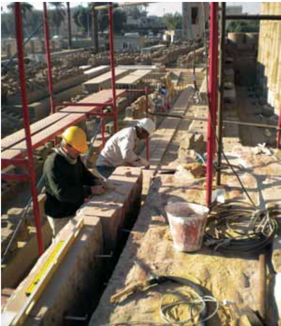
Amenhotep III outer wall slabs being mortared into place
