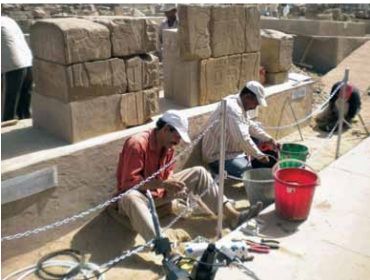
Sami and Saber installing lamps in the blockyard open-air museum
