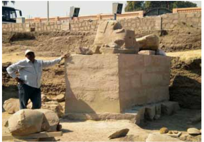
Sphinx being restored on sphinx road
