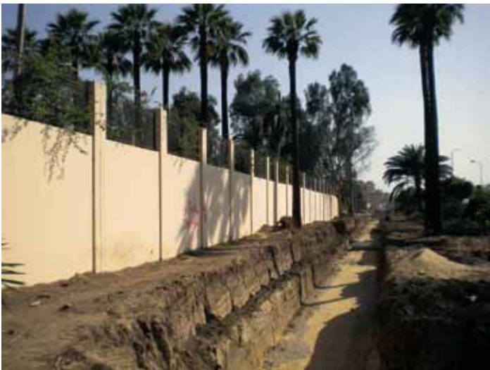
Service tunnel trench outside Chicago House, March 24, 2010
