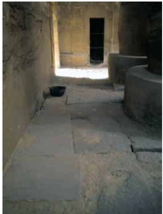
Khonsu Temple court ambulatory new floor blocks in place after documentation
