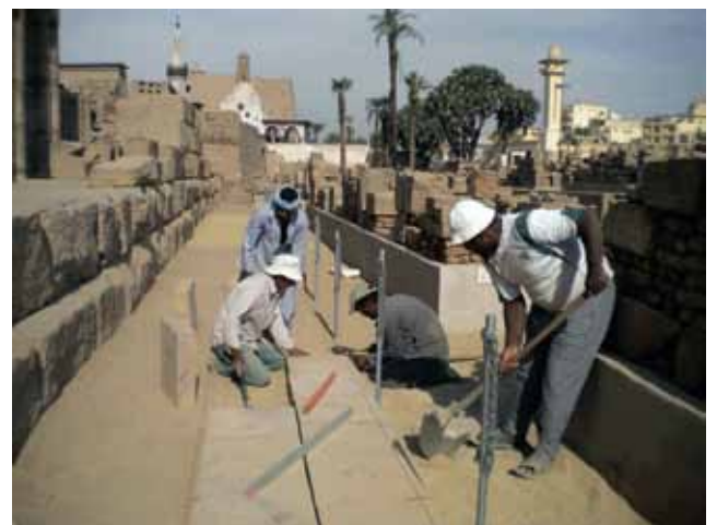
Luxor Temple blockyard open-air museum path construction
