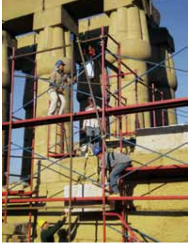
Amenhotep III outer wall slab construction
