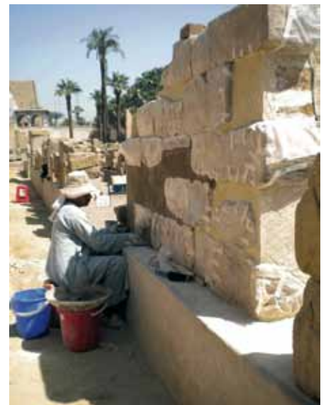
Alaa plastering the infilled surface of the Nectanebo group
