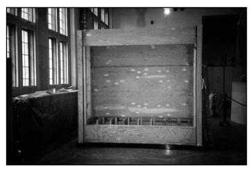
View of west side of new exhibit case that will feature heavy funerary reliefs; at this stage of construction, reinforced deck and space for recessed lights are prepared
