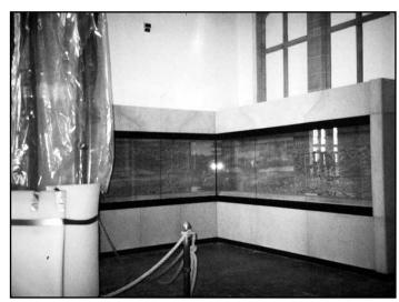
Completed chronology case with limestone sheathing and glass doors, which are specially designed without dividers; floor of case sits above angled ramp for labels
