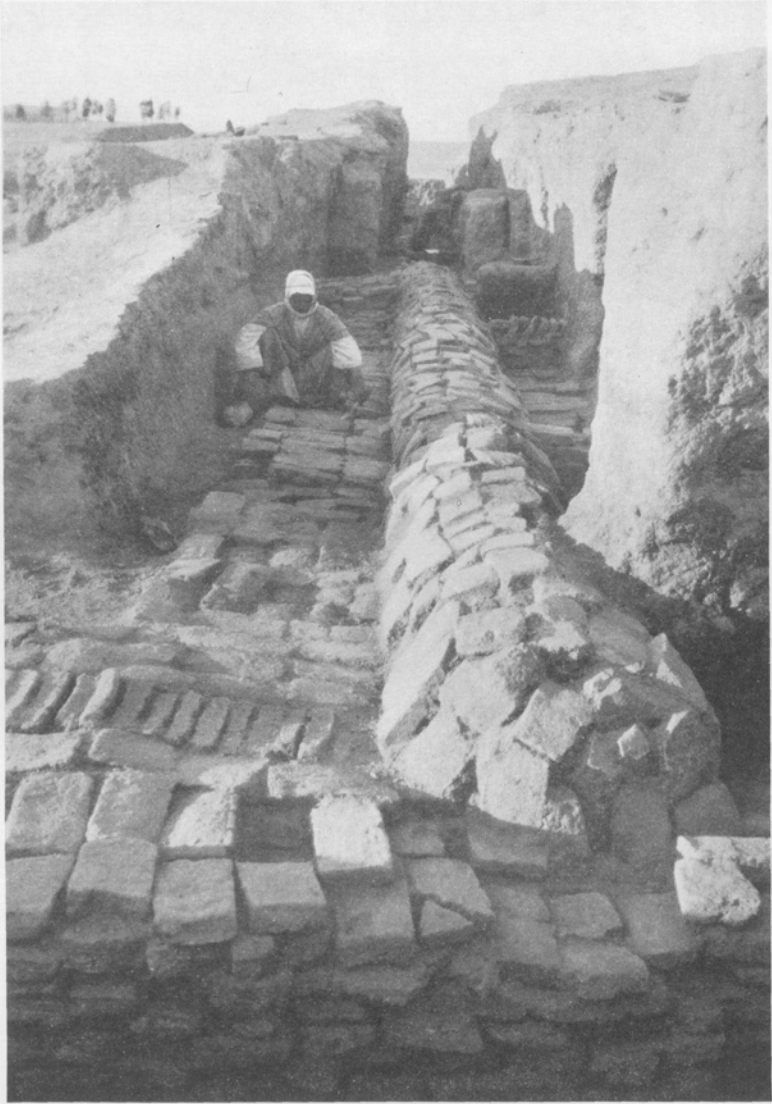
FIG. 26.—Upper end of palace sewer, with drain from a bathroom entering from left.
