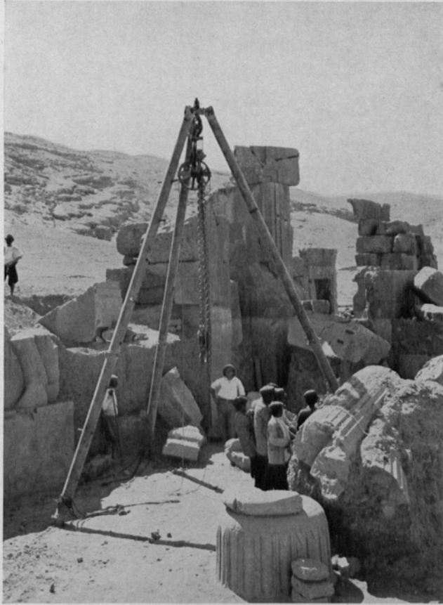
FIG. 66.—Removing stones in the northern portico of the Hundred-Column Hall.
