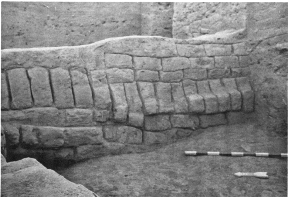
Fig. 17.—Area WA, Square 12, revetment Wall F from the west. Note the irregular construction of very large mud bricks.
