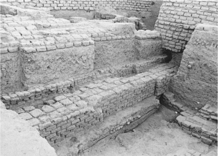
Fig. 8.—Area WA, Square 12, Wall L running under Wall K, from the east
