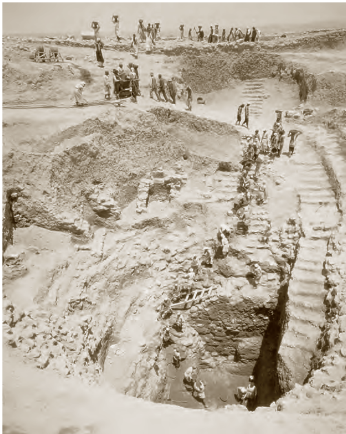
FIGURE 7.6 The excavation of Megiddo, 1931 (OIM Megiddo field negative A460)
