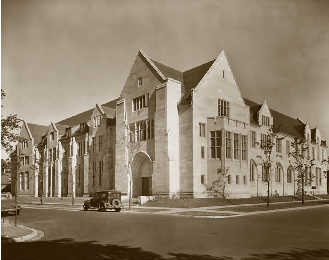
FIGURE 7.18 The Chicago headquarters of the Oriental Institute, opened in 1931. The building contains laboratories, offices, a reference library, museum preparation areas, storage, 16,000 square feet of museum galleries, an auditorium, and two small classrooms (OIM photograph P. 18730)
