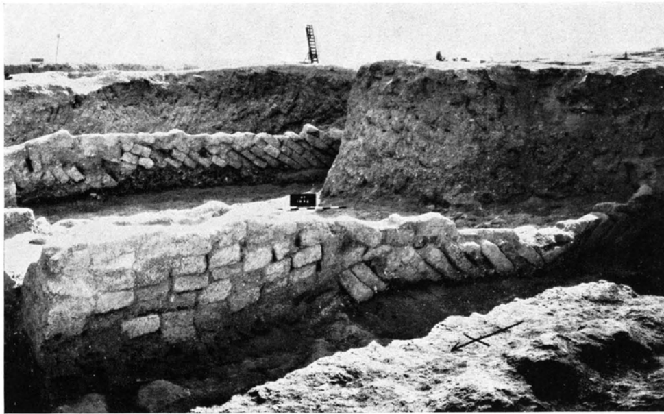
FIG. 41.—MUD-BRICK REINFORCING WALLS IN FILLING BELOW STABLE COURTYARD
