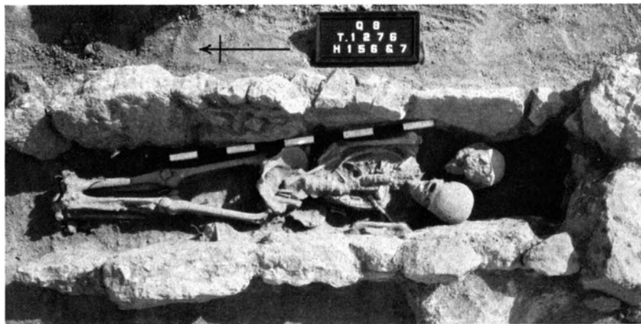
FIG. 110.—TOMB 1276 WITH COVER SLABS REMOVED
