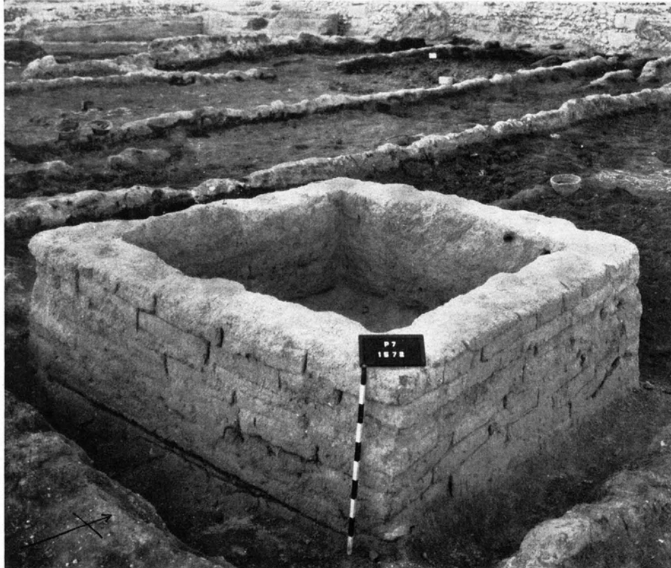
FIG. 42.—MUD-BRICK WATER TANK NEAR CENTER OF STABLE COURTYARD
