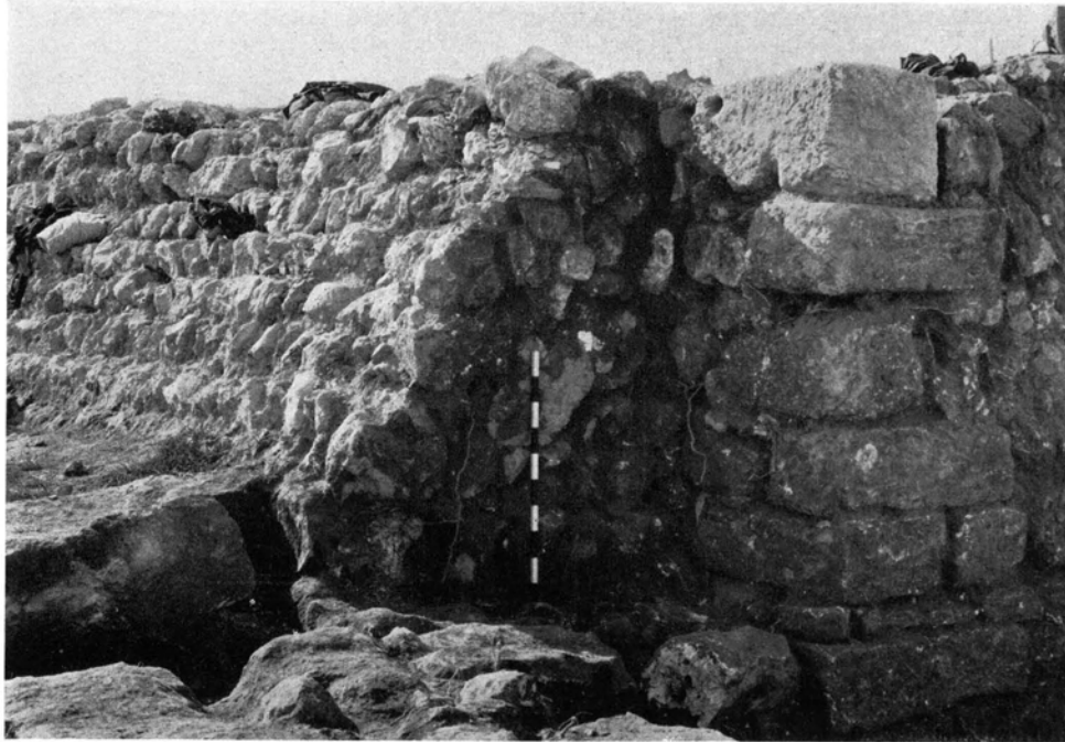
FIG. 81—NORTHEAST CORNER OF ROOM 575 IN BUILDING 1052 , SHOWING REUSED STABLE PILLAR AND BATTERED REVETMENT WALL 971
