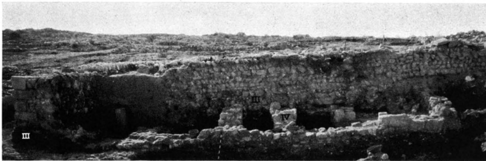
FIG. 83.—FOUNDATION OF BUILDING 1052 , FROM NORTH
