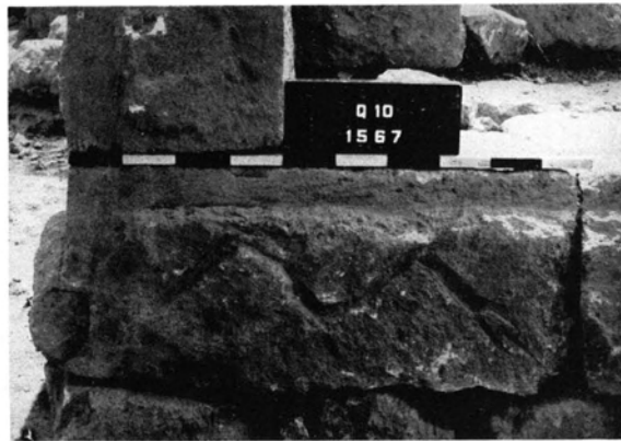
FIG. 16.—NORTHEAST DOORJAMB OF GATEWAY, SHOWING MASON'S SETTING-OUT MARK (IN LOWER LEFT CORNER) AND HIS IDENTIFICATION MARK
