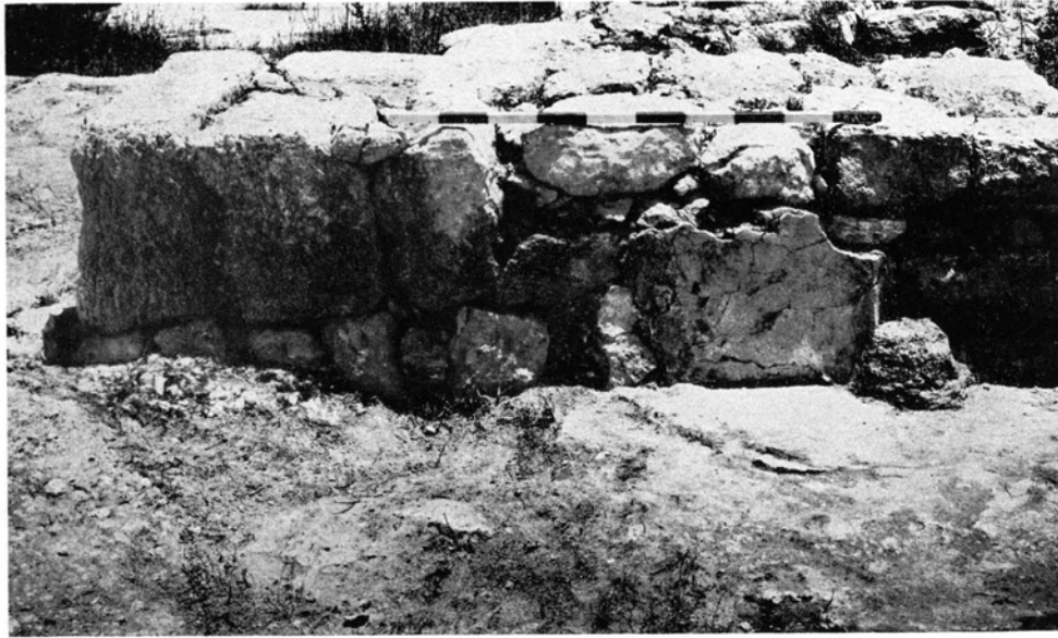
FIG. 45.—PLASTER ON FRONT EXTERIOR WALL OF STABLE UNIT 403. POSSIBLY REMAINS OF A ROOF DRAIN
