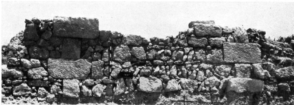
FIG. 13.—DETAIL OF MASONRY IN EAST WALL OF STRATUM IV B INCLOSURE, FROM WEST
