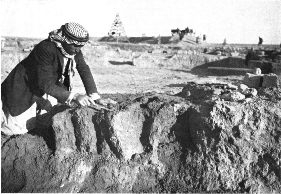
FIG. 91.—MUD BRICKS PLACED ON EDGE TO RAISE THE FLOOR LEVEL OF THE AUDIENCE HALL, IN DOORWAY BETWEEN P 27:1 AND P 27:8
