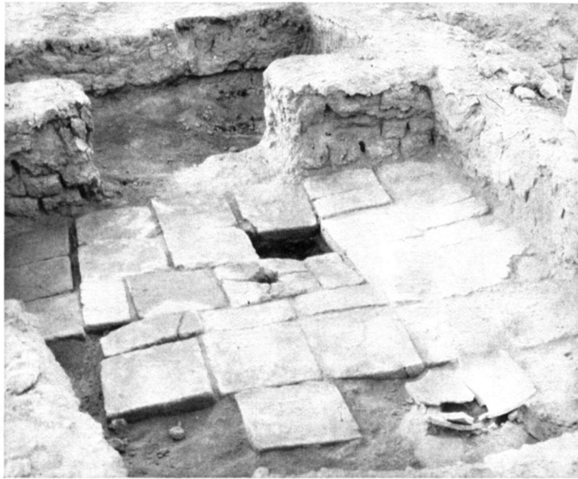
FIG. 80.—PAVEMENT OF IBIQADAD I BRICKS IN A PRIVATE HOUSE (IN Q 33:14) BENEATH THE SOUTHERN BUILDING, SHOWING PIERCED BRICK IN CENTER; SEEN FROM EAST
