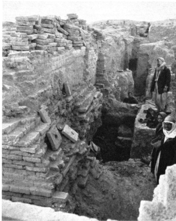
FIG. 54.—CLEARING AWAY THE BRICKWORK IN ENTRANCE (M 32:8) AND ENTRANCE VESTIBULE (M 32:7), SEEN FROM SOUTHEAST
