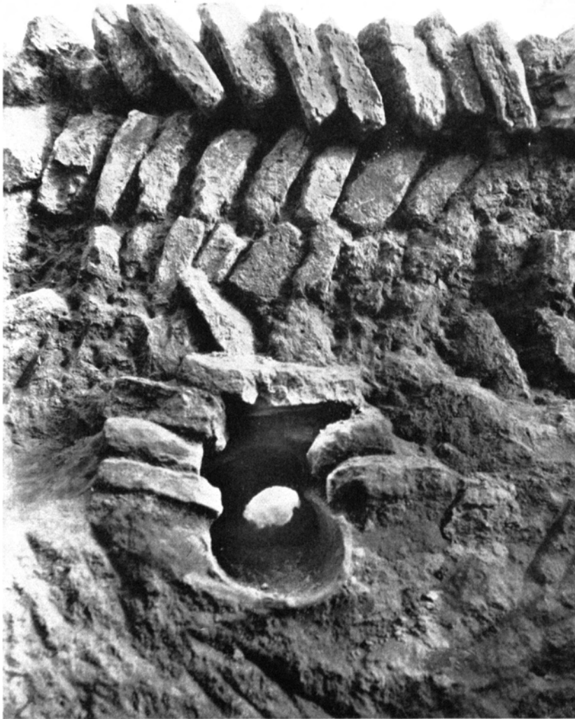
FIG. 112.—TUBULAR POTTERY DRAIN REINFORCED BY BAKED BRICKWORK, LEADING THROUGH THE OUTER INCLOSURE WALL IN J 44
