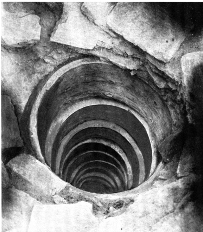
FIG. 113.—DEEP VERTICAL SHAFT M 44:8 (CF. PL. III), FORMED BY A SERIES OF TUBULAR POTTERY SECTIONS
