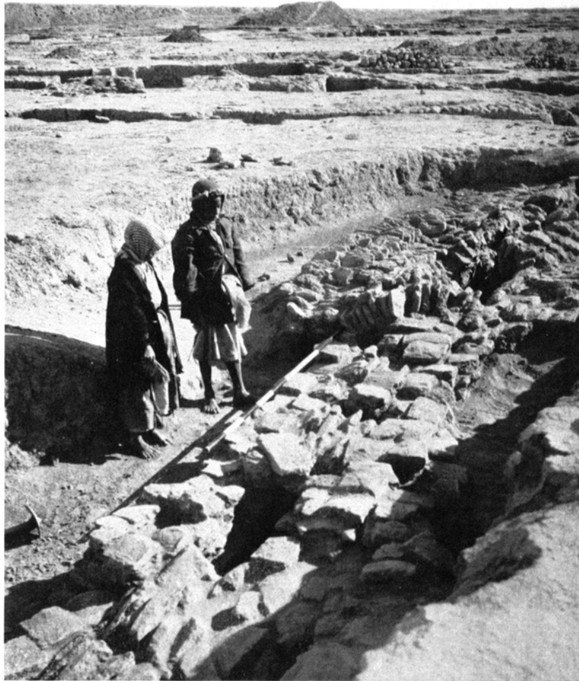
FIG. 116.—DETAIL OF THE COVERING OF THE LARGE VAULTED DRAIN K 46:8
