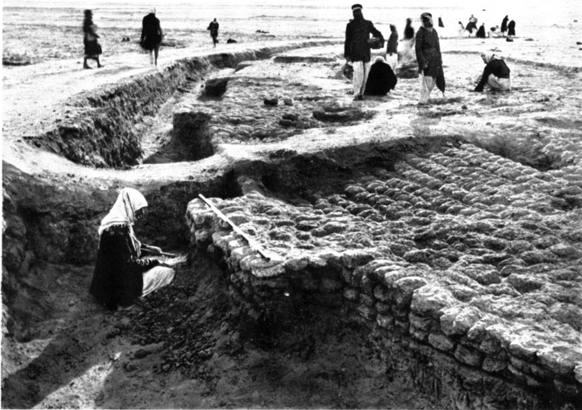
FIG. 66.—THE BUTRESSES OF THE OUTER INCLOSURE WALL ON THE EAST SIDE
