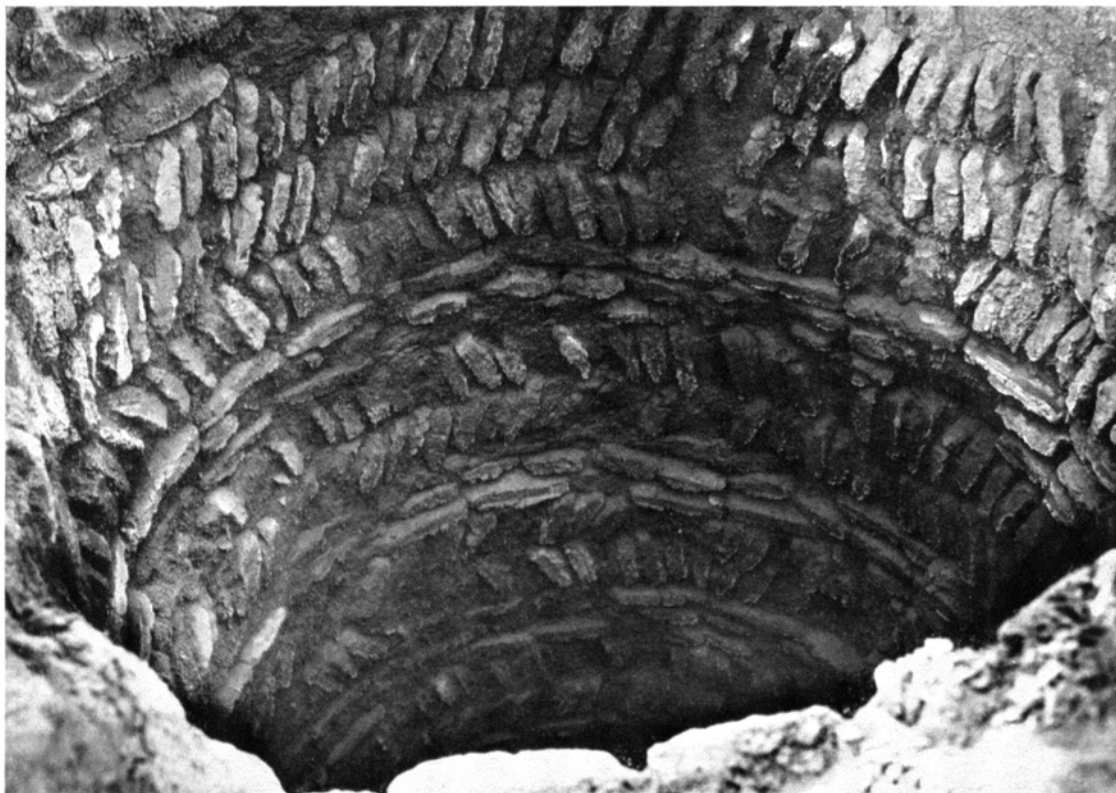
FIG. 109.—THE BRICKWORK OF WELL L 45:2
