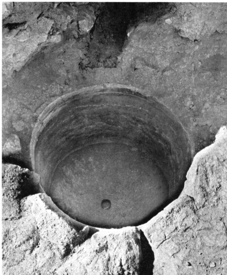
FIG. 114.—FUNNEL-SHAPED VERTICAL DRAIN AT THE END OF THE HORIZONTAL DRAIN OUTSIDE M 43:1
