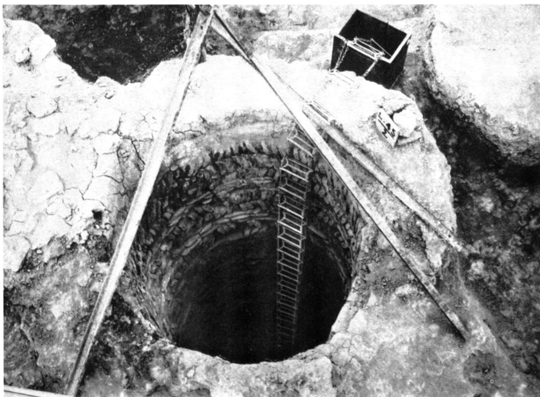
FIG. 34.—THE WELL L. 45:2 IN THE COURTYARD
