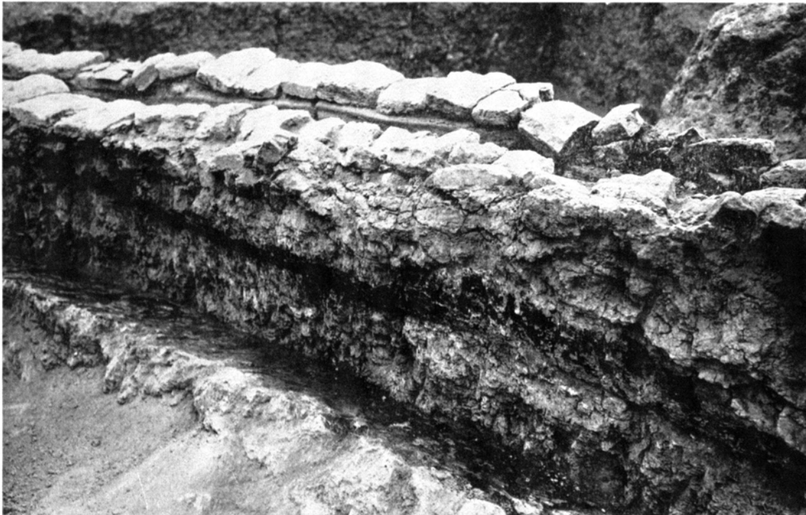
FIG. 111.—BAKED BRICKS USED IN THE CONSTRUCTION OF THE DRAIN IN K 46:4
